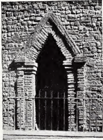
107. HOLY TRINITY, COLCHESTER. SAXON DOORWAY
